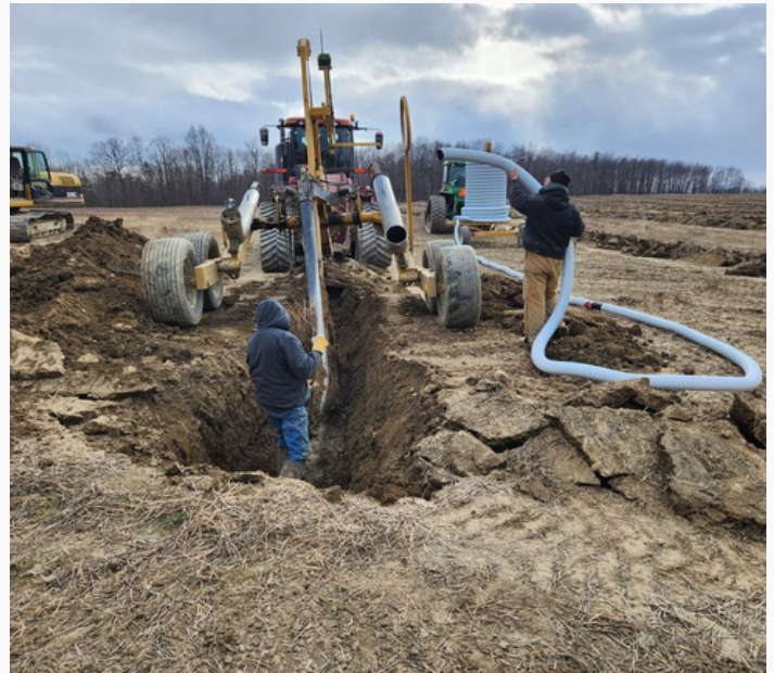
Workers install a culvert at Tommy Creek in Lodi
